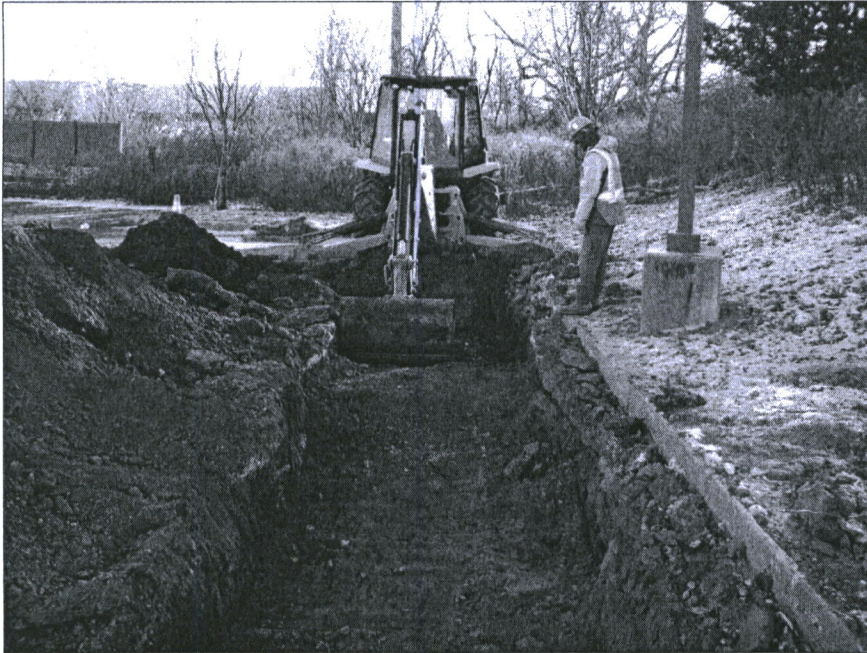
Figure 9. 100 Sockanosset Cross Road west trench, view east.
