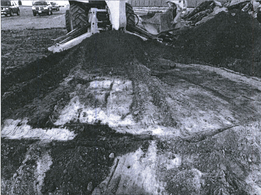
Figure 7. Asphalt and topsoil removal work in progress, view north.
